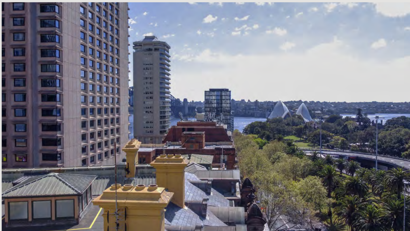
Existing site photo - No.317, Victoria Parade - upper level
