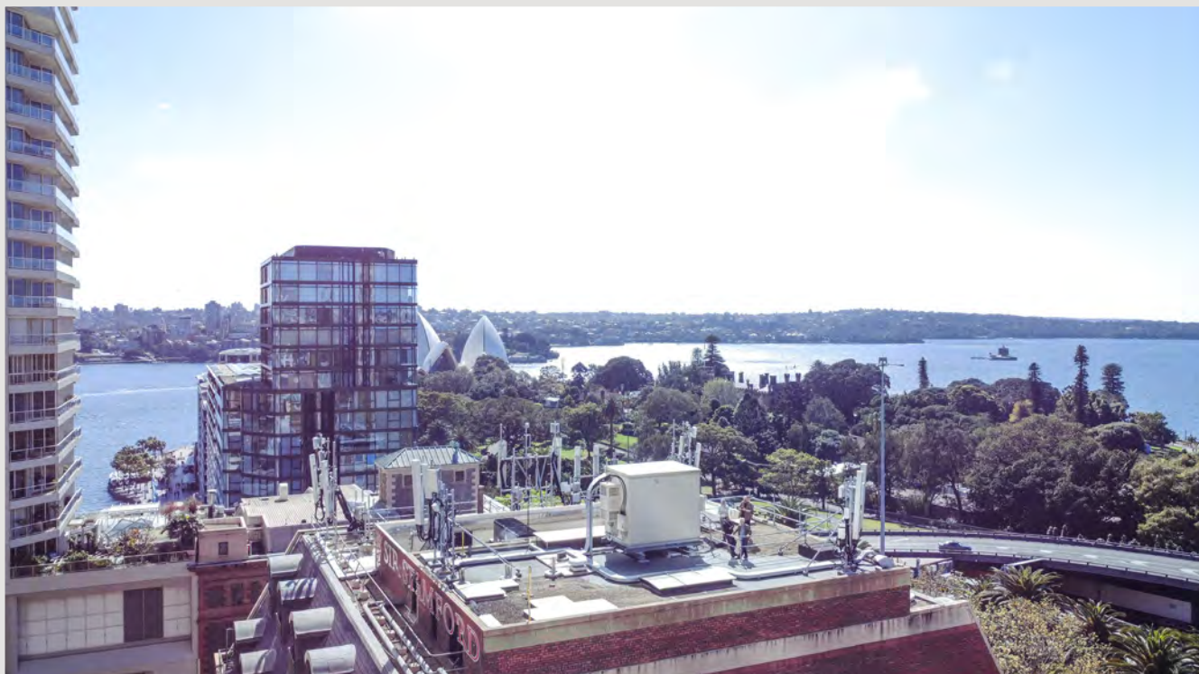
Approximate site photo - InterContinental Hotel
