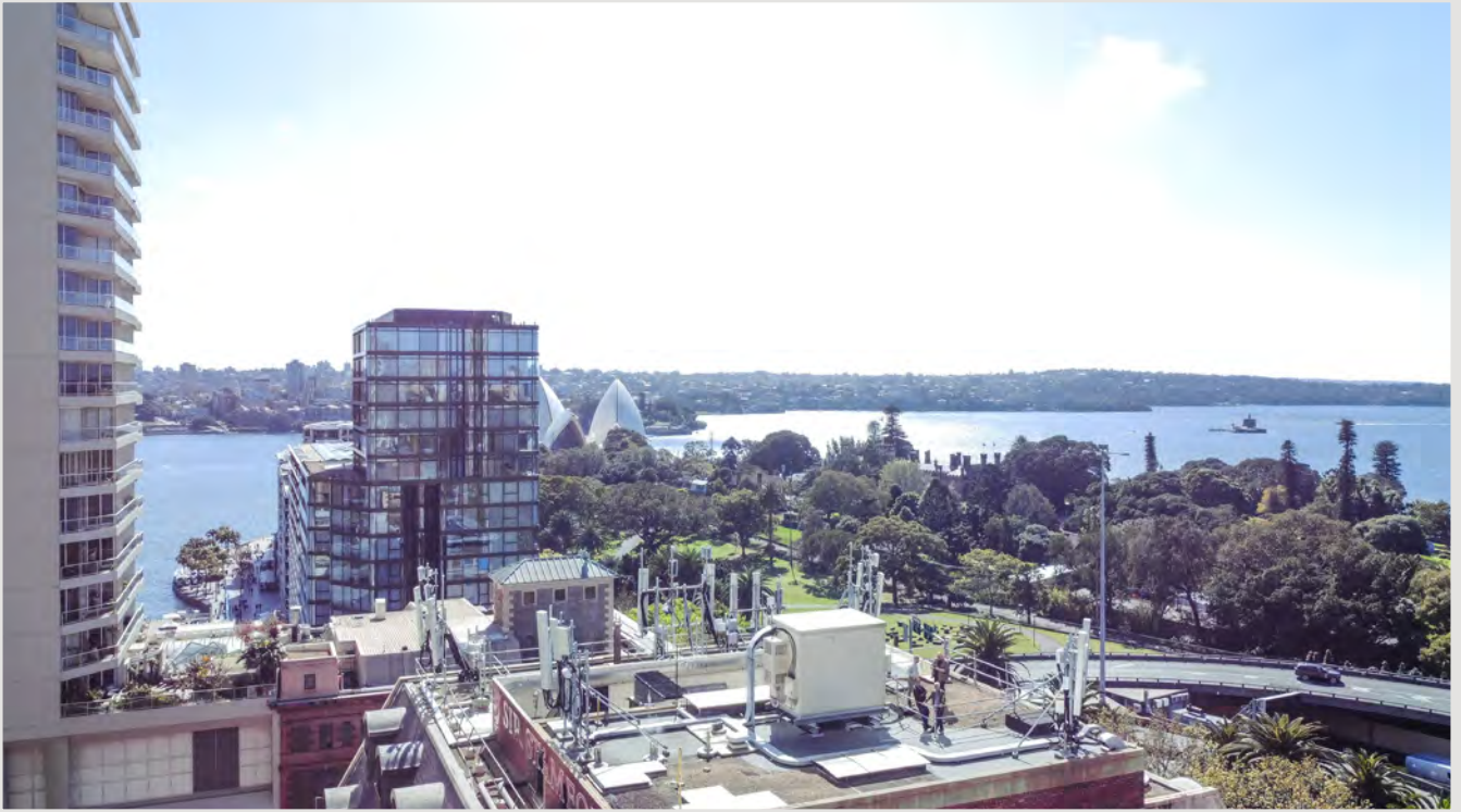
Approximate site photo - InterContinental Hotel
