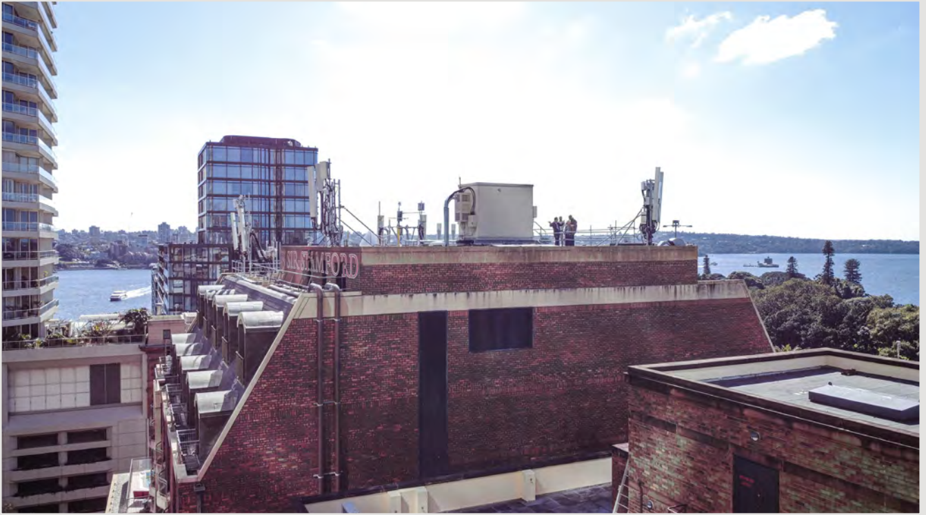
Approximate site photo - InterContinental Hotel
