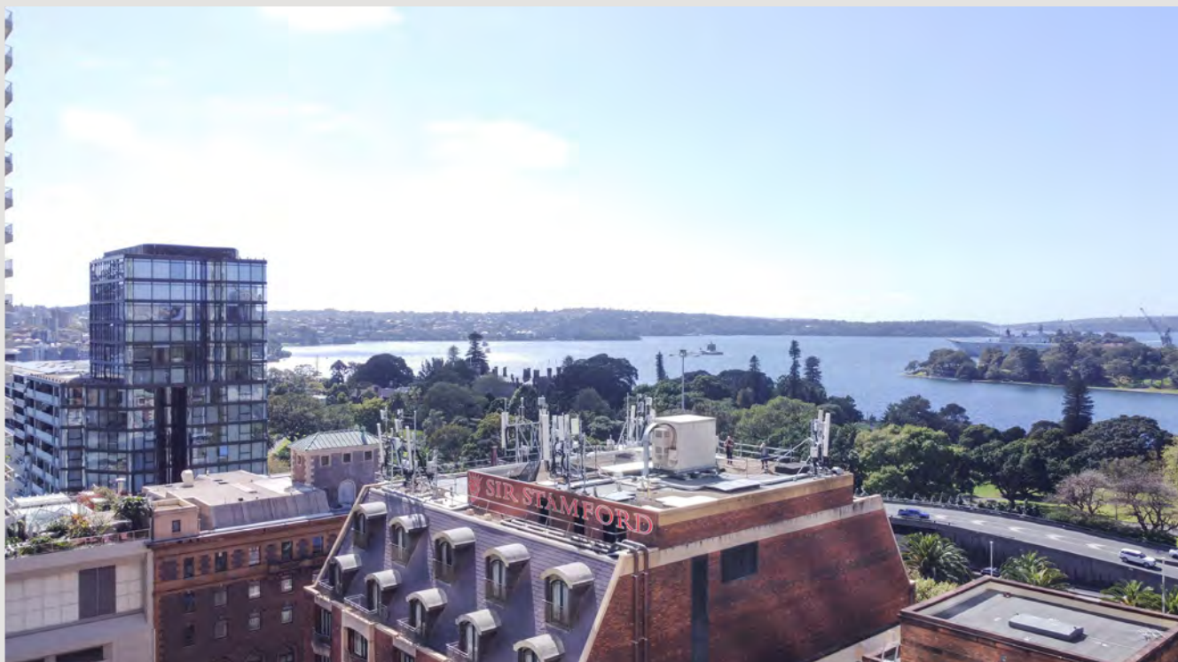
Approximate site photo - InterContinental Hotel
