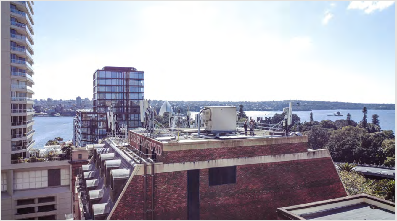
Approximate site photo - InterContinental Hotel
