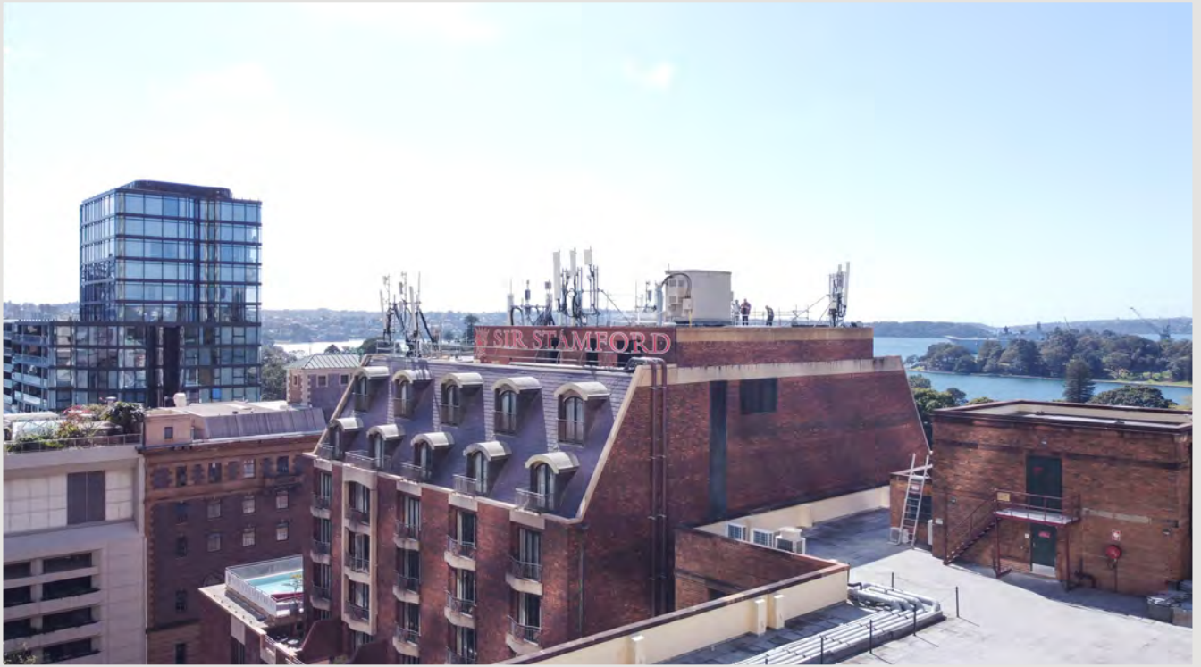
Approximate site photo - InterContinental Hotel
